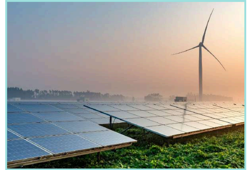
Figure C1 | Wind turbine and solar panels example.
