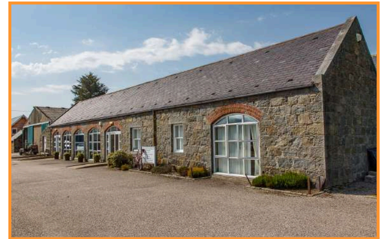
Figure Fiiib | Netherton Rural Business Centre , Aberdeenshire
